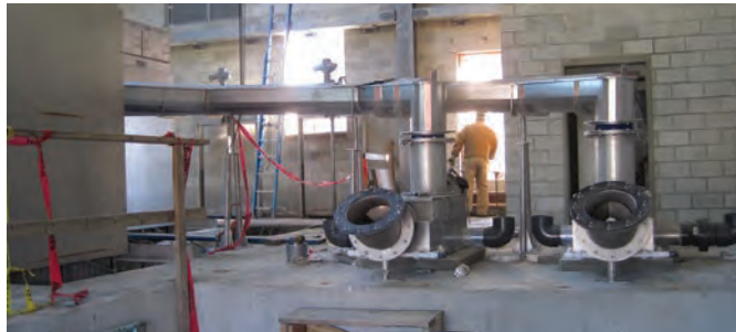
Common sluice able to isolate duty/standby Whitetip Shark Washing Compactor.
